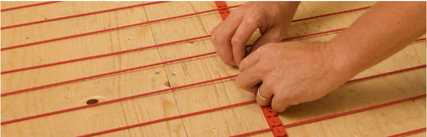
FIGURE 2.29: Install stabilizing guides
