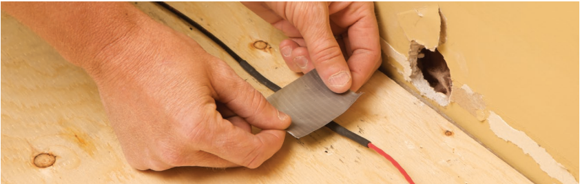
FIGURE 2.23: Secure the cold lead to the subfloor
