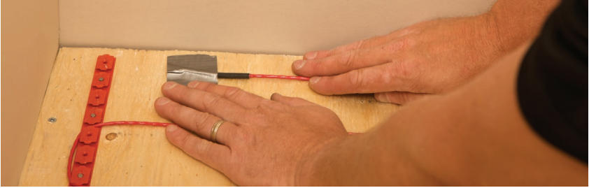
FIGURE 2.28: Secure the end seal
