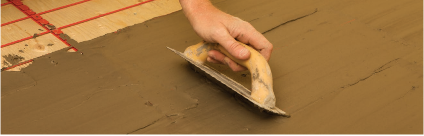
FIGURE 2.52: Thinset mortar method
