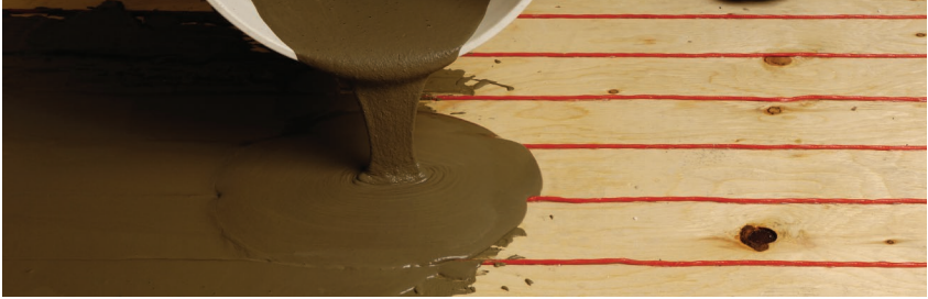
FIGURE 2.42: Self-leveling compound method
