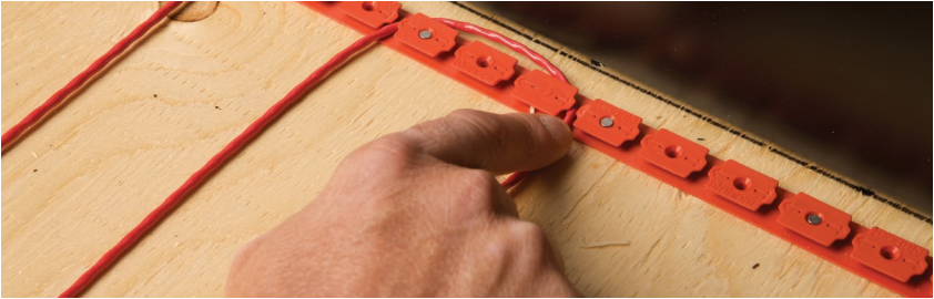
FIGURE 2.26: Install the heating cable
