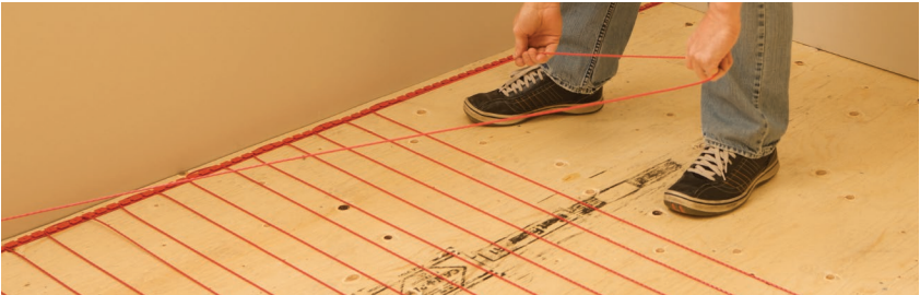
FIGURE 2.27: Install the heating cable
