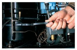
The FreezGard crankcase heater's self-regulating design automatically varies heat output to maintain adequate oil temperature, while minimizing energy use.
