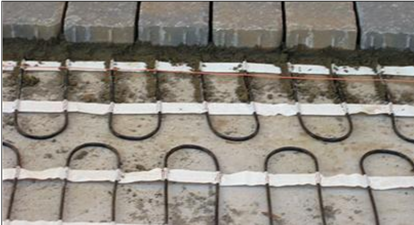
Example of proper compacted depth on cables.
