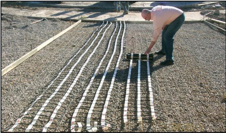
Rolling out the heating mat prior to the concrete pour.
