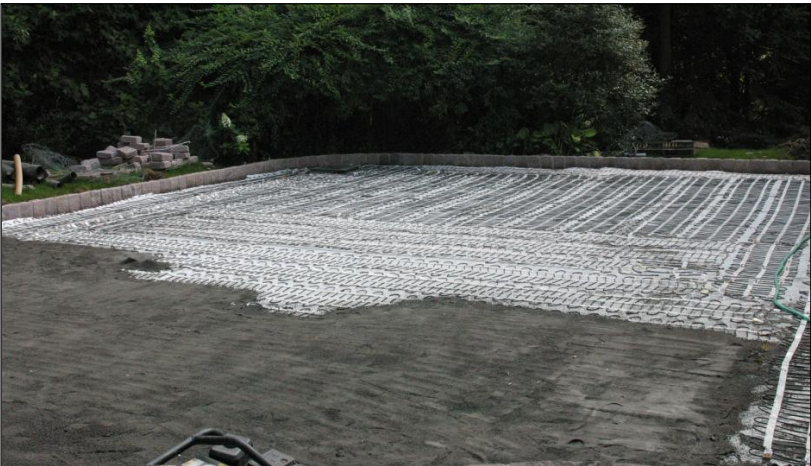
Paver sand being applied over snow melting mats.
