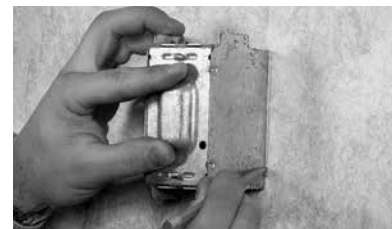
Figure R5. Marking outline on wall
