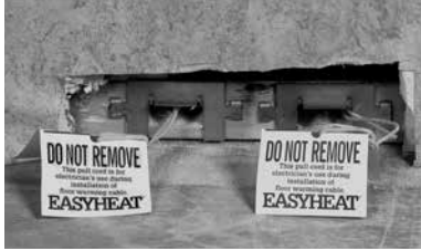
Figure R6. Fish cord installation
