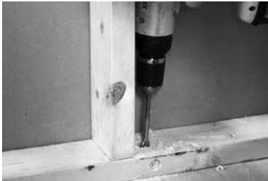
Figure N4. Fish hole preparation
