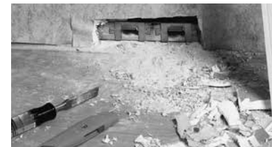
Figure R4. Fish hole clearing
