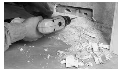
Figure R3. Fish hole preparation
