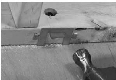
Figure N5. Guards installation
