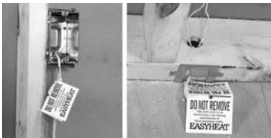
Figure N7. "Do Not Remove" tags installation
