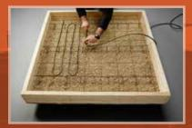
Use the included twist ties to secure the heating cable to a properly installed welded wire mesh or rebar reinforcing system.
