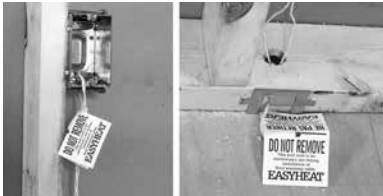
Figure 1c. “Do Not Remove” tags installation
