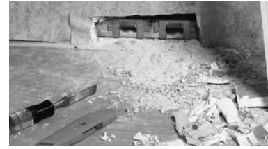
Figure 1e. Fish hole clearing
