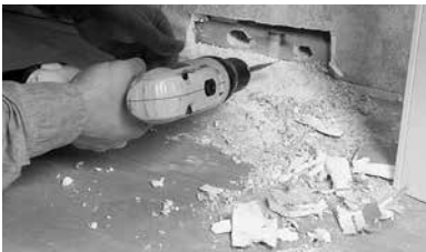
Figure 1d. Fish hole preparation
